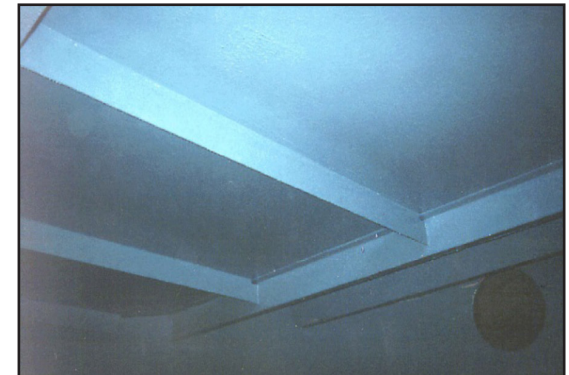
Roof and top of silo completed
