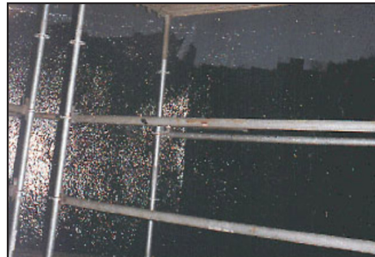
First coat of ARC 855 being applied
