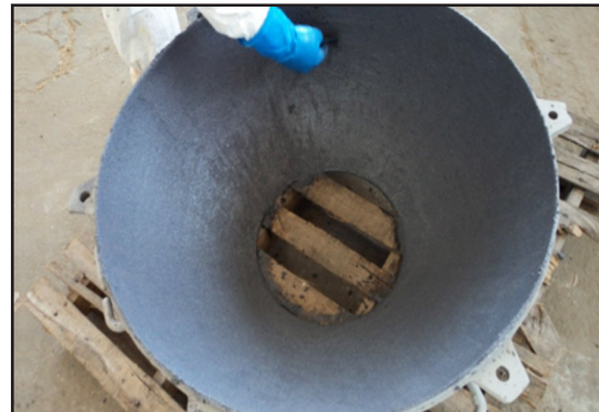
Application of ARC coatings
