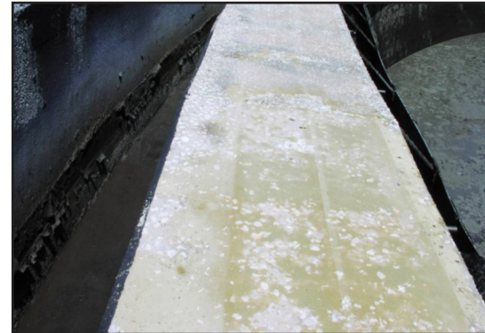
Surface cleaned and damaged concrete removed
