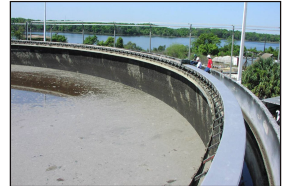
ARC 791 being applied with screed box
