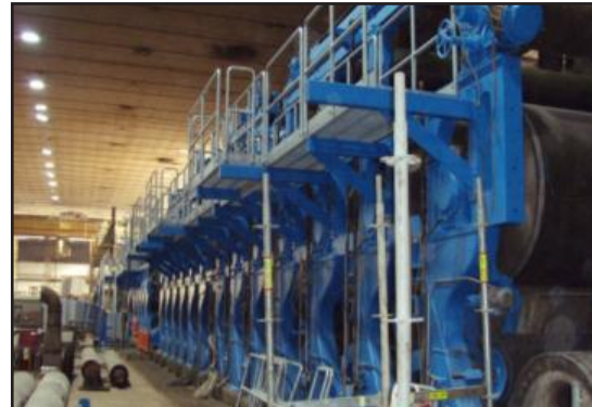
ARC S1PW applied to frame during refurbishment
