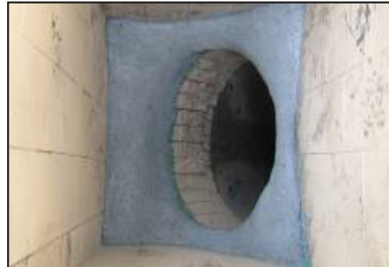
Installation of ARC MX5
