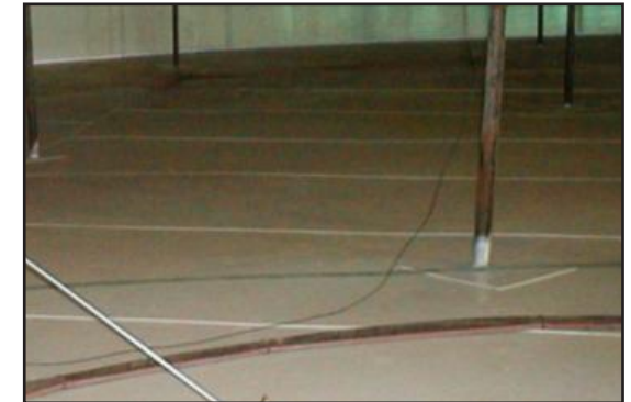
Final inspection of the ARC lining to ensure a continuous pinhole free protective lining
