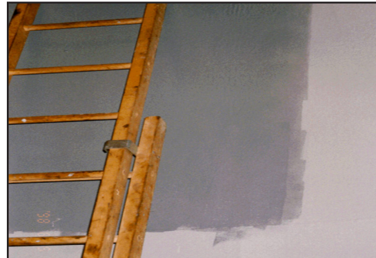
First coat of ARC S7
