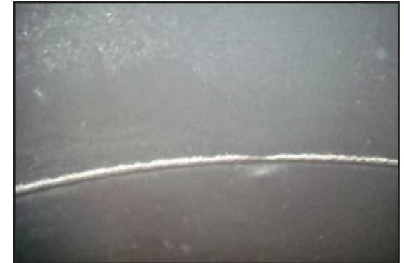
ARC S7 lining still in excellent condition after 10 years of service
