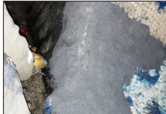
Applying ARC IBX1
