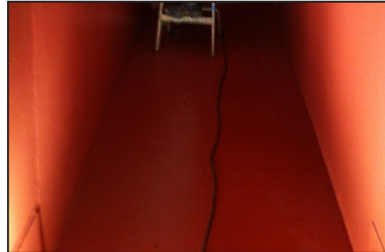
ARC S7 is applied in ducts using airless spray equipment
