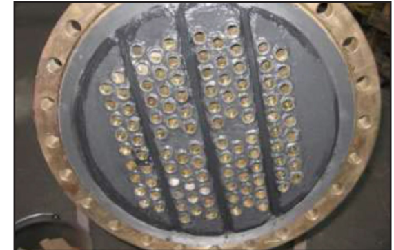
Completed tube sheet
