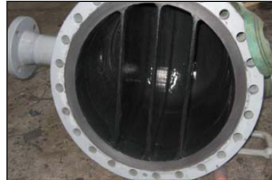
Repaired divider plates
