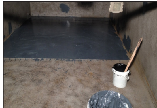
Applying ARC 858 to resurface and fare smooth pitted surface
