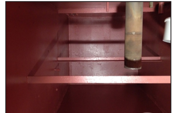
Completed tank internals
