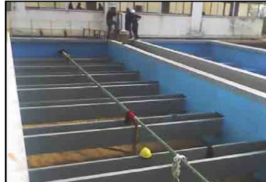
Installing ARC S1PW coating
