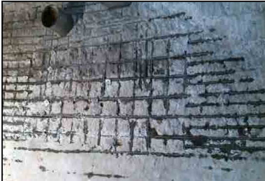
Chest wall after tile removed and blasted
