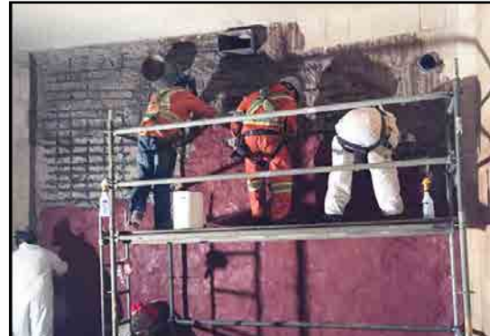
Installing ARC NVE coating
