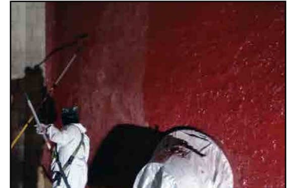
Applying NVE sealer coat
