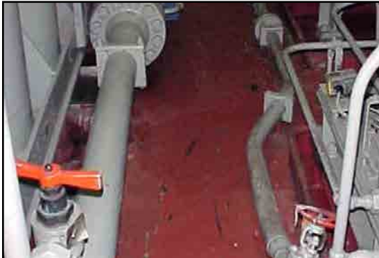
Existing coating 1 year after installed
