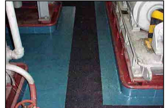
High traffic regions coated with ARC 855N for non-slip
