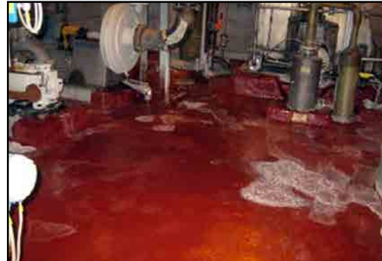
ARC NVE VC in service
