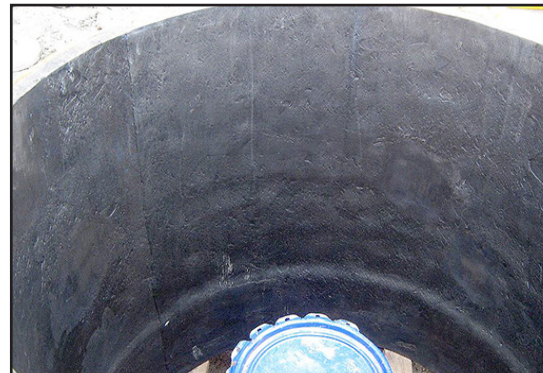
Rubber surface is prepared by roughening with flapper wheel.
