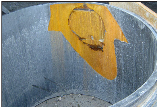
External metal patch welded on chute to extend MTBR.
