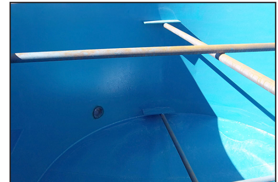
Tank bottom half after application of 2 coats of ARC SD4i
