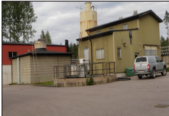
Wet well location.
