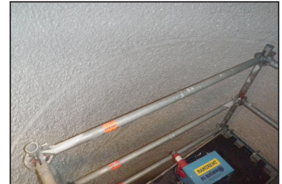
Surface of the wet well with final coat of ARC S1HB .
