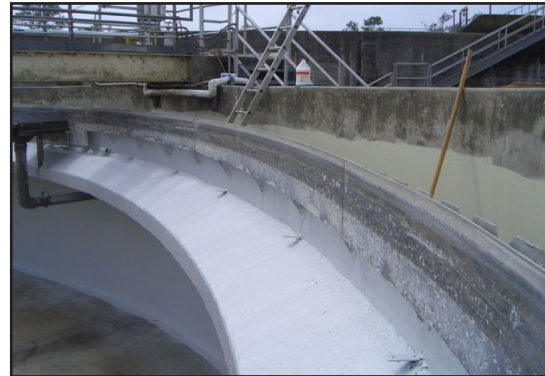
In the process of applying ARC S1HB
