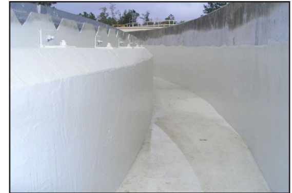
Final finish applied to clarifier
