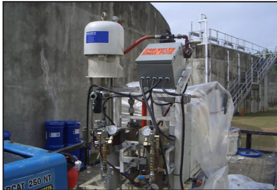
Heated plural component used to apply ARC S1HB
