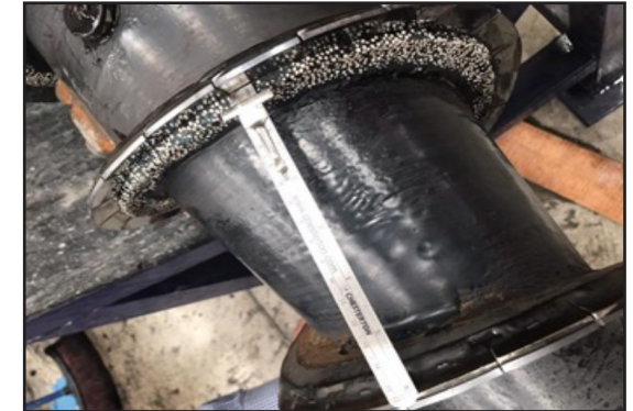
The final coat of ARC SD4i on stay vanes.
