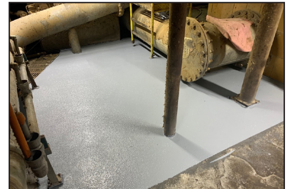
ARC EG-1 with tight ARC CS2 finish coat.
