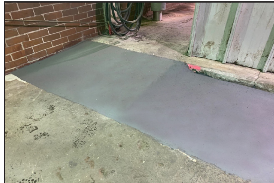
Sloped ramp reconstructed or repaired.
