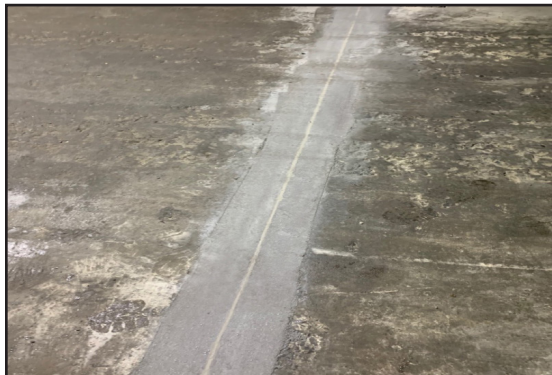
Damaged expansion joints rebuilt with ARC EG-1.
