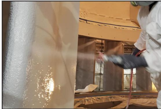
Plural component spraying of ARC S1HB up to 150 mils in a single coat.
